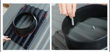
**Step 3** Cut out the marked "D" shape using hacking knife, tin snip or nibbler.
