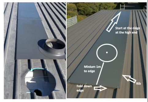
the lower pieces by a minimum of 100mm. All joints to be properly sealed and pop riveted.
