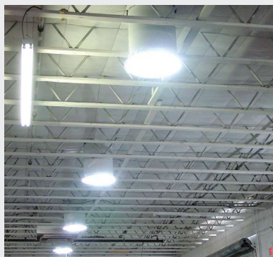
Warehouse Open Ceiling
